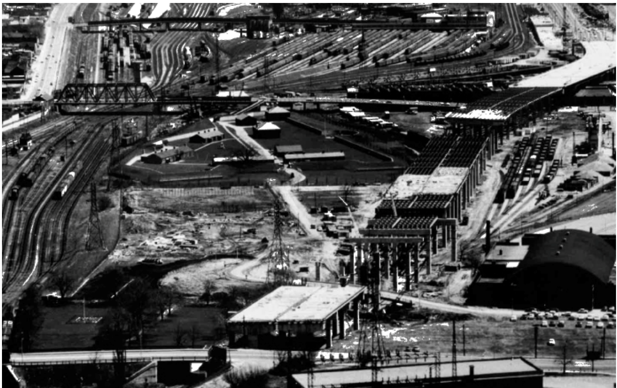
Plate 4: Gardiner Expressway under construction by Fort York in 1960, looking east. Note ground surface change and construction facilities over the former Ordnance and Supply Yard area in the centre of the photo.
