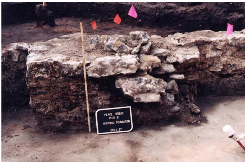
Plate 4.4: The limestone and chert block foundation in Pier 2—detail of the fireplace.
