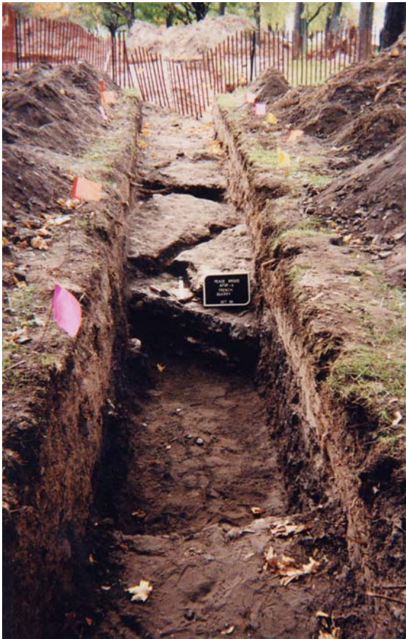
Plate 4.7: View towards the quarry face exposed in the NPC Building water/sanitary sewer trench.
