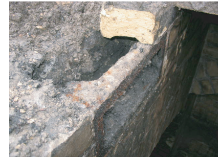
(d) View of the southeast chamber. Note that a course of bricks has been removed from the arch and the interior face of the pier and the areas resurfaced with mortar.
