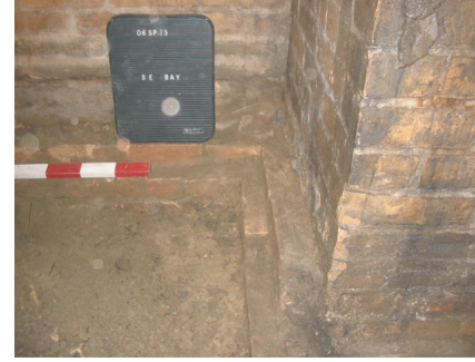
(c) Exposed pier footing between the south end and southwest bays.
