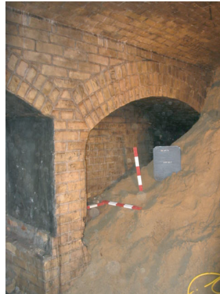
(f) View of the northwest chamber partially choked with sand fill used to block the entry.
