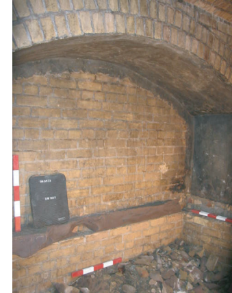
(d) View of the southeast chamber. Note that a course of bricks has been removed from the arch and the interior face of the pier and the areas resurfaced with mortar.
