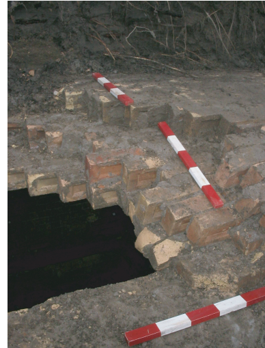
(e) Detail of the construction of the barrel vaulted roof.
