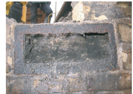
(h) Views of the ventilation flue in the south end of the mausoleum.
