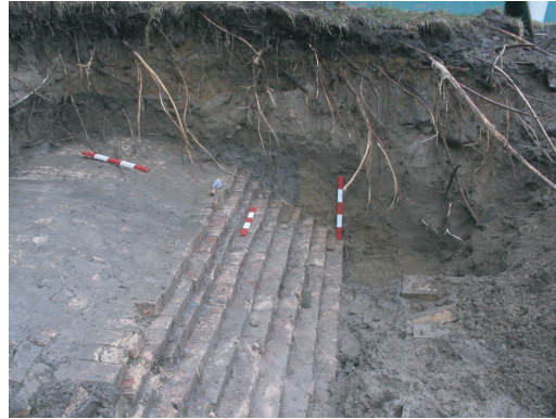
(b) View of the corbelled courses of brick rising to the crown of the vaulted roof.
