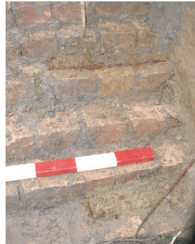
(d) Detail of iron staples incorporated into the brickwork. Their placement corresponds to the location of the interior pier between the interior arches on the east wall of the north chamber. No staples were used in the corresponding location on the east wall of the south chamber.
