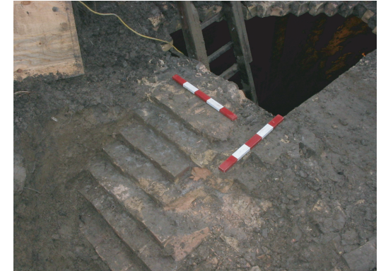
(f) View of damage to the corbelled courses of brick at the southeast corner of the structure that likely resulted from the construction of the 1920s house.
