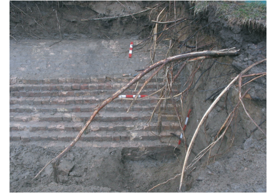
(c) View of the corbelled courses of brick rising to the vaulted roof and the uppermost course of the wall.
