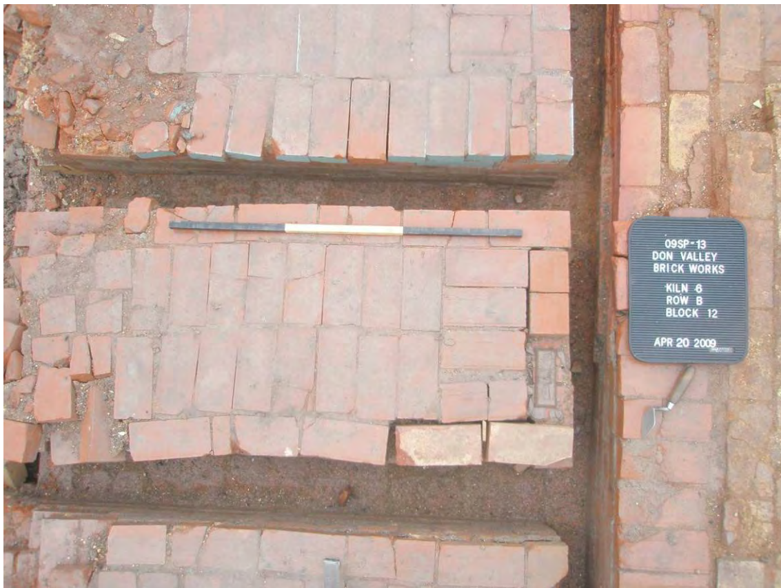
Plate 10: Detail of one of the blocks between the floor channels showing the diverse range of bricks, in this case including enameled specimens, used in the construction/repair of the kiln base.
