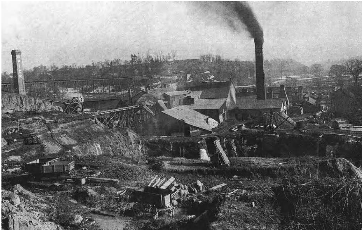
Plate 11: The brick works operations in the 1890s, viewed from the northwest. Note the series of chimney stacks behind and to the right of the “Don” chimney, which appear to be the rectangular downdraught kilns. Toronto Reference Library, Baldwin Room SC128.
