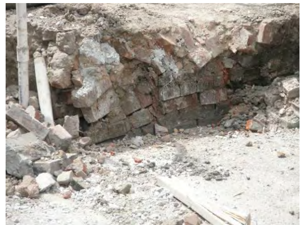
Plate 34: Exposure of a Building 11C footing in the south part to the Crane Pad excavation area.
