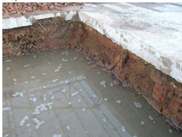
Plate 46: Exposure of a portion of Kiln 13 under the floor of Building 14. Note the rubble filled void of the flue at the upper left of the photo.
