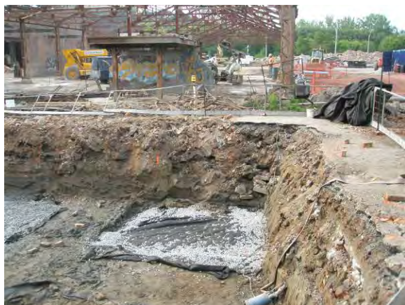
Plate 31: View of the remains of the Building 11B brick walls in the south face of the Pedestrian Bridge excavation area.
