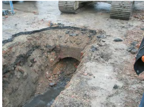
Plate 29: The initial exposure of the top of the possible Kiln 5 chimney draw hole chamber in the 1500mm watermain trench near Fire Hydrant 5.
