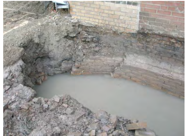
Plate 48: View of the flue at the base of the wall of Building 9 where it begins to turn north to connect to Kiln 9.
