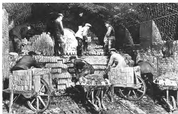
Plate 9: Cleaning up a down-draught kiln at the Don Valley Brick Works following a flood, 1920. Photo courtesy of E. Freeman.
