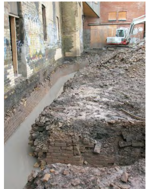
Plate 48: View of the flue at the base of the wall of Building 9 where it begins to turn north to connect to Kiln 9.
