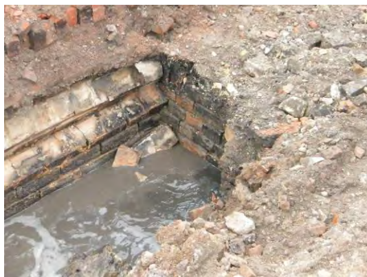
Plate 43: The central flue of Kiln 6. To the right (north) of the brick wall built across the conduit, the flue had been decommissioned at the time of demolition. The wall was then installed to close off this break in the system.
