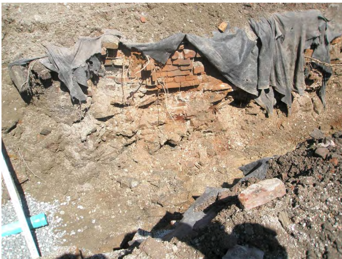
Plate 8: Exposure of the shale and concrete slab perimeter foundation of Kiln 6 during the service installations carried out after the Stage 4 documentation.
