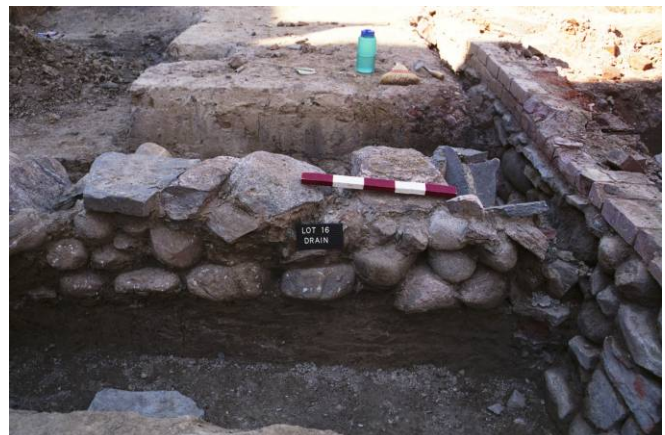
Plate 15: East end of stone box drain (Lot 16) where it is truncated by addition to Townhouse 4, looking north.
