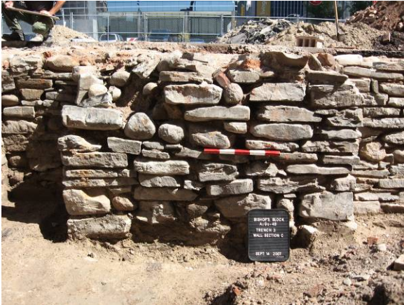
Plate 20: Stone fireplace foundation on west wall of Townhouse 3 rear basement room.
