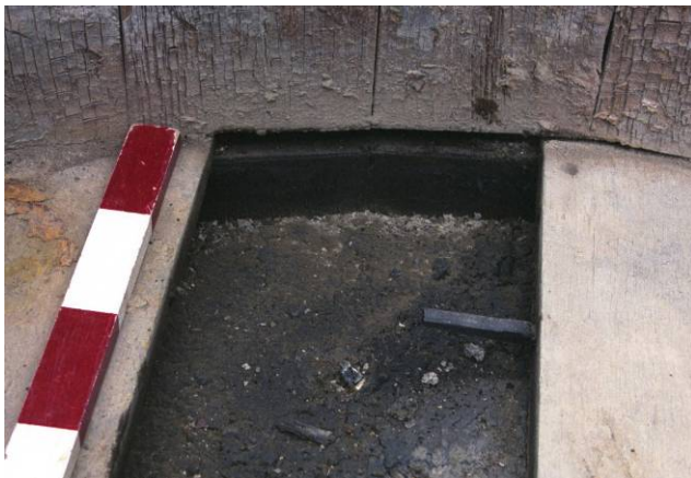
Plate 10: Close up of wooden peg used in Cistern 2 construction.
