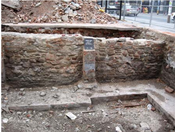
Plate 24: Looking east across concrete floor with sump depression in the basement of Townhouse 4.
