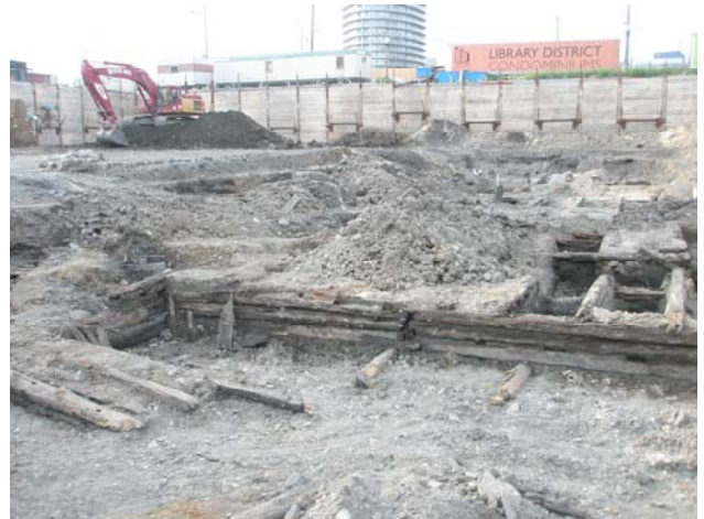
Plate 32: The north limit of the interior cells of the cribbing, defined by a plank clad wall on the northwest side of the structure. Note the runners underlying the entire structure extending beyond the wall.
