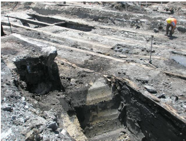
Plate 9: Bulk heavy clay lake fills (Lot 90) on the east side of the Queen's Wharf lying on lake bed sediments.
