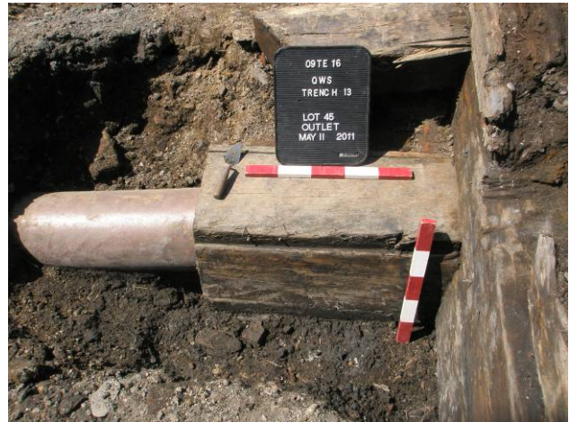
Plate 20: View of the ceramic drain on the south side of the engine house entering the wood box conduit through the Garrison Creek west crib wall (Lot 45 drainage system).
