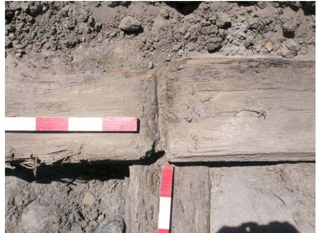
Plate 36: An example of poor construction practice in the form of an unfastened butt joint directly above a mortise and tenon, creating a natural weak spot. This indicates that the cribbing was not required to withstand extreme lateral forces.
