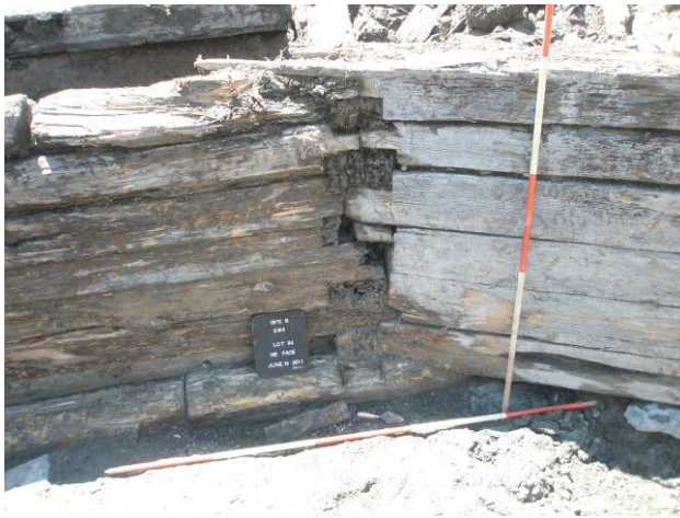
Plate 31: Complexly beveled mortise and tenon joinery required to accomplish the widening of the crib structure.
