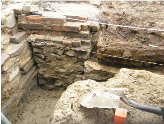
Plate 55: View of the limestone footing underlying the Lot 33 forge/machinery base and Lot 34 bin.
