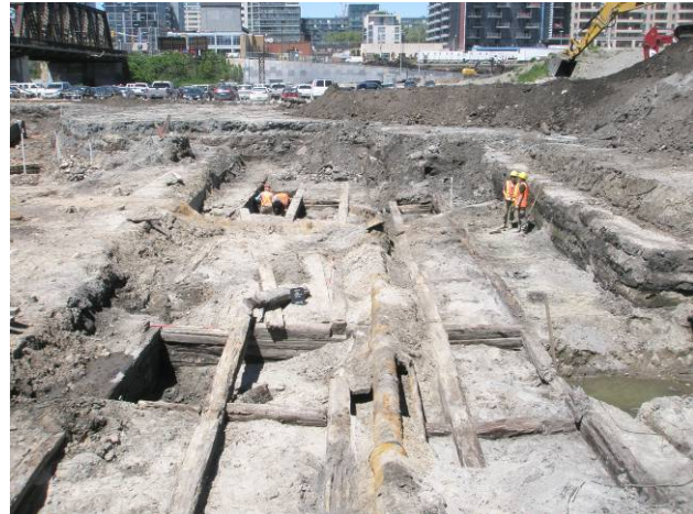
Plate 24: View of the south portion of the landbound portion of the Queen's Wharf structure (Lot 64). The large cast iron pipe running along the top of the structure is a later gas main (Lot 73).
