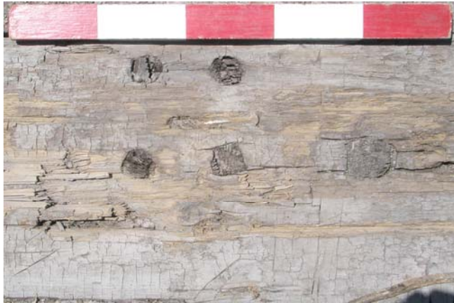
Plate 35: Relic tree nails that have been trimmed flush to the face of the beam. These have no function in the Queen's Wharf structure built by the GTR and so indicate reuse of timbers.
