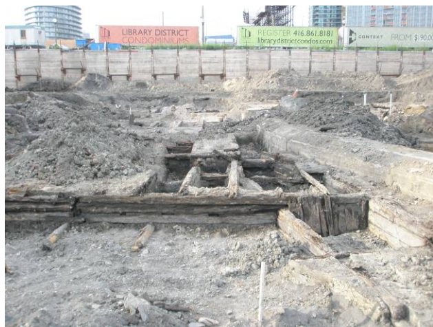
Plate 33: The north limit of the interior cells of the cribbing, defined by a plank clad wall on the northeast side of the structure. Note the runners underlying the entire structure extending beyond the wall and the lateral runners laid under and to the west of the east exterior wall.
