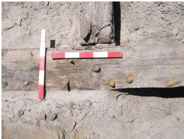
Plate 25: Remnant decking nails and a tree nail securing a mortise and tenon tie back on the upper surface of the crib structure.
