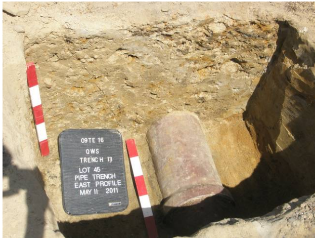
Plate 19: View of a section through the trench cut-and-fill for the installation of the ceramic drain on the south side of the engine house (Lot 45 drainage system).
