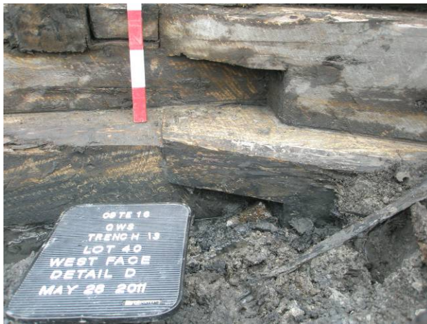
Plate 13: View of the lap joinery used to accomplish the turn of the east Garrison Creek crib wall.
