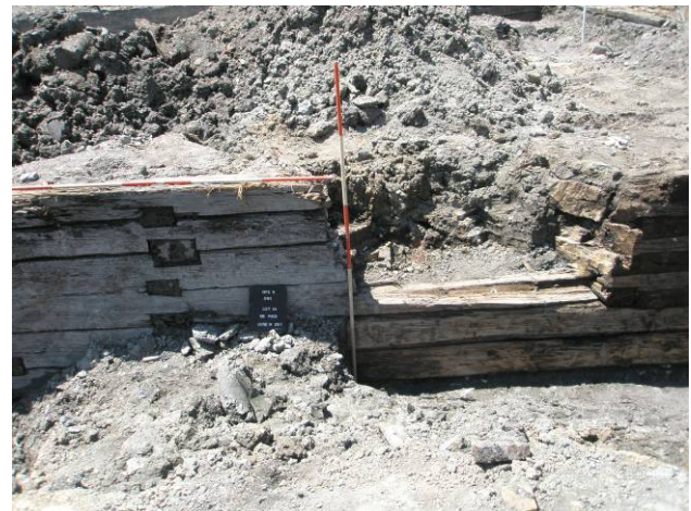
Plate 26: A section of the east exterior wall of the crib structure cut away for the installation of a later valve chamber (Lot 101).
