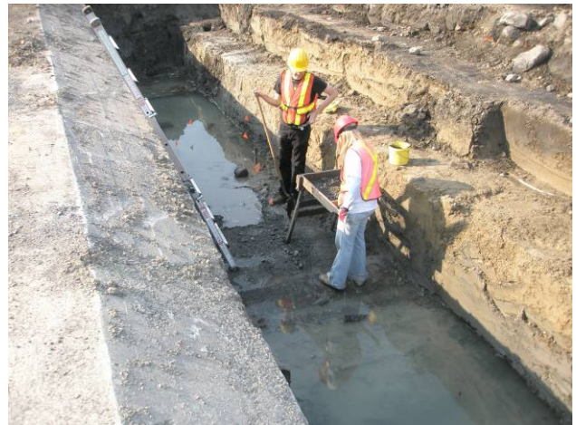
Plate 8: Bulk heavy clay lake fills (Lot 90) between Garrison Creek and the Queen's Wharf lying on lake bed sediments.
