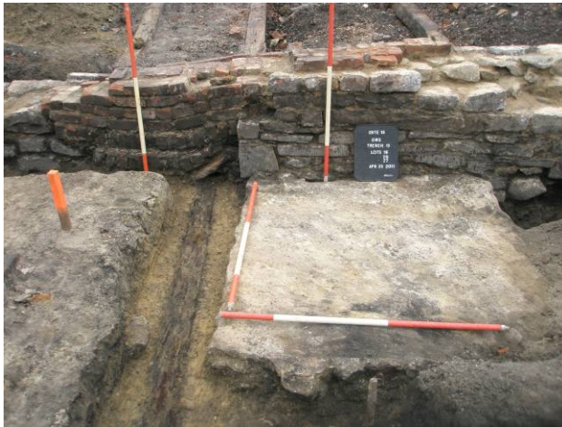
Plate 43: Lot 25 equipment footing/base in plan from the south. A later utility installation (Lots 14/27) through the foundation of the GTR engine house is to the left of the masonry feature.
