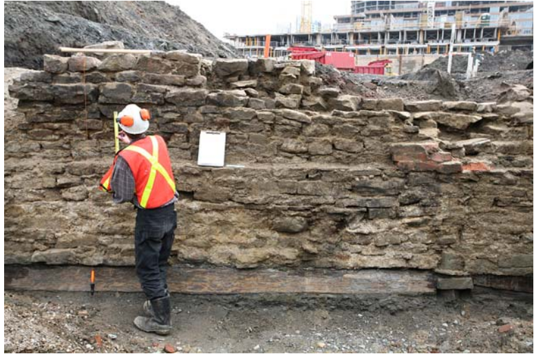
Plate A1-2: East foundation of GTR engine house standing on original nearshore lakebed materials.
