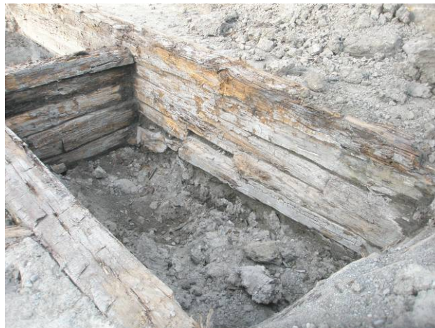
Plate 29: View of the articulation of an interior tie back wall (upper left) and the west exterior face wall (right). The timber in the lower left is a single beam saddled on top of the tiebacks.
