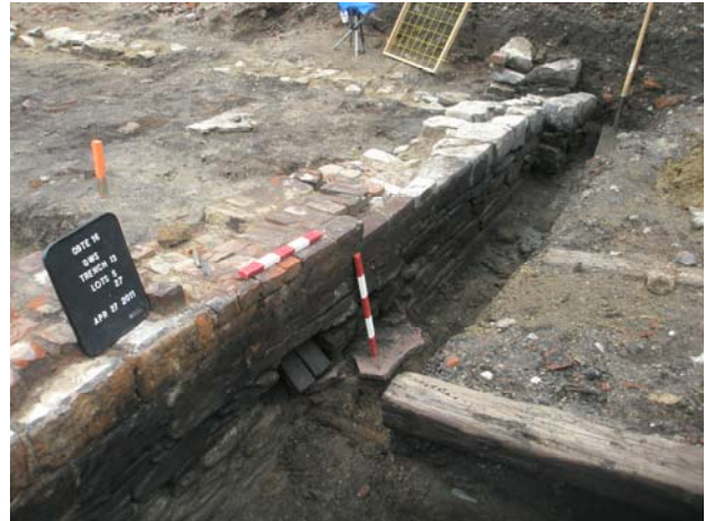
Plate 48: Lot 27 brick repair work to the north foundation wall of the GTR engine house required following the installation of the Lot 14 cast iron utility pipe to the building, viewed from the north (exterior).
