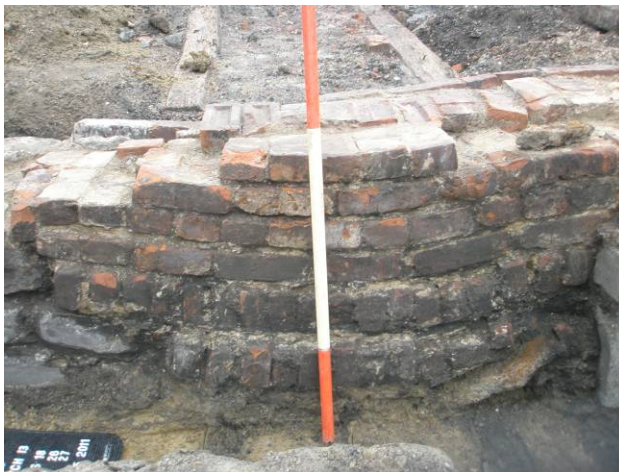
Plate 49: Lot 27 brick repair work to the north foundation wall of the GTR engine house required following the installation of the Lot 14 cast iron utility pipe to the building, viewed from the south (interior).
