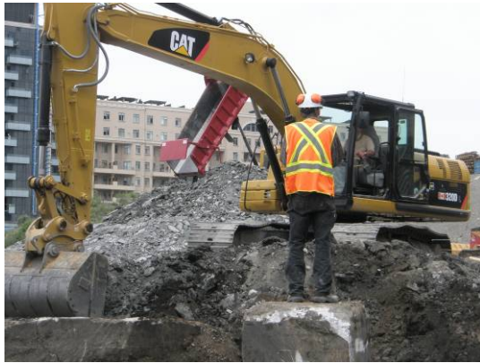
Plate 1: Mechanical removal of fills.
