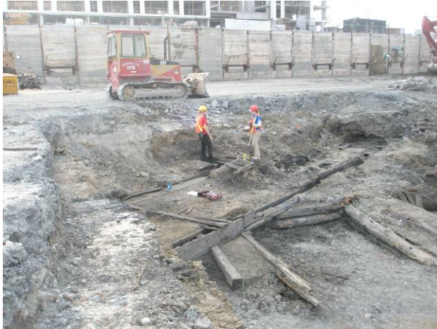
Plate 27: A network of box drains (Lots 80-82) cutting through the extreme northeast corner of the crib structure.
