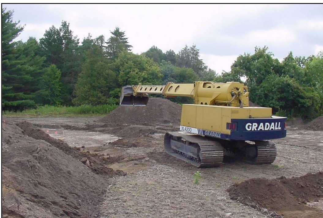
Plate 4: Mechanical topsoil removal at the McNair site.
